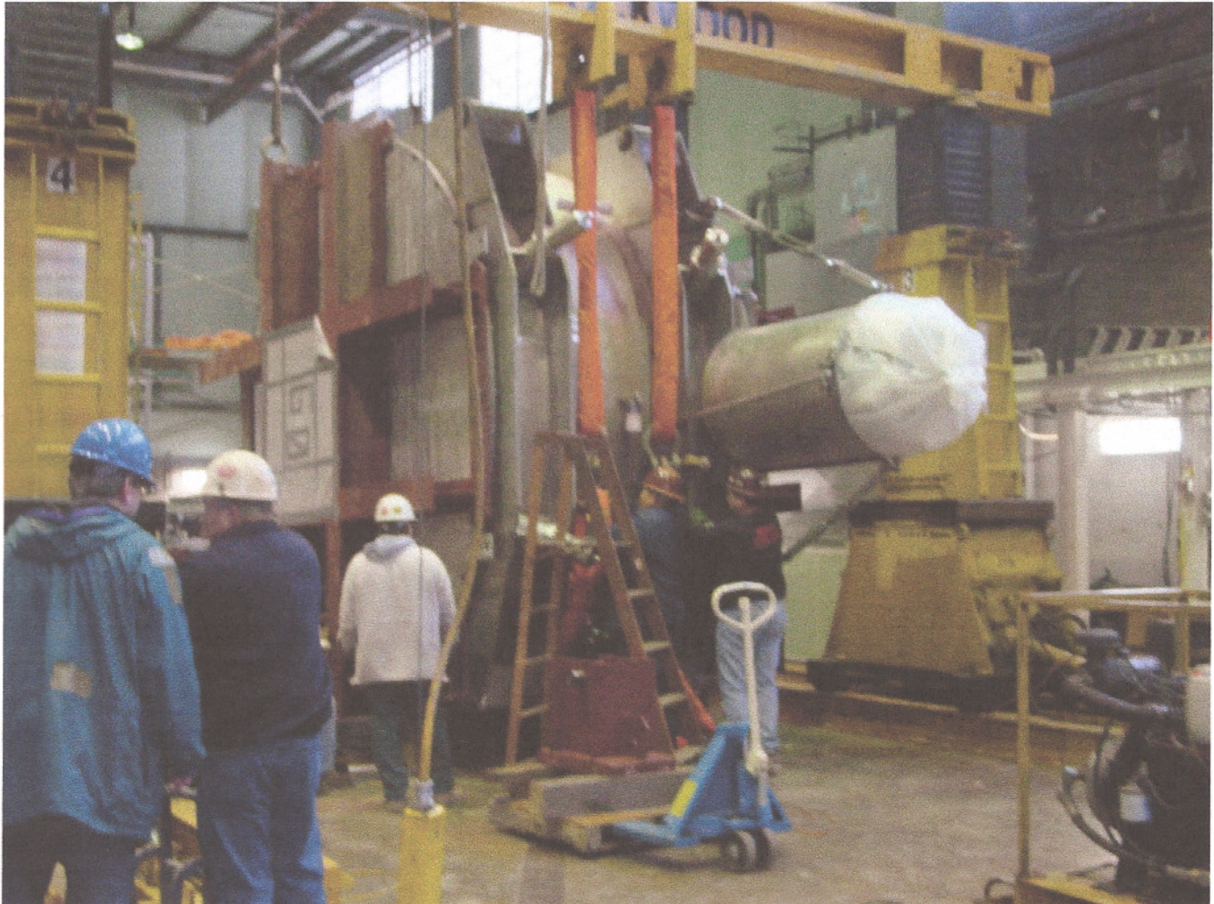
Photo 5 Installing Feet in Illinois
