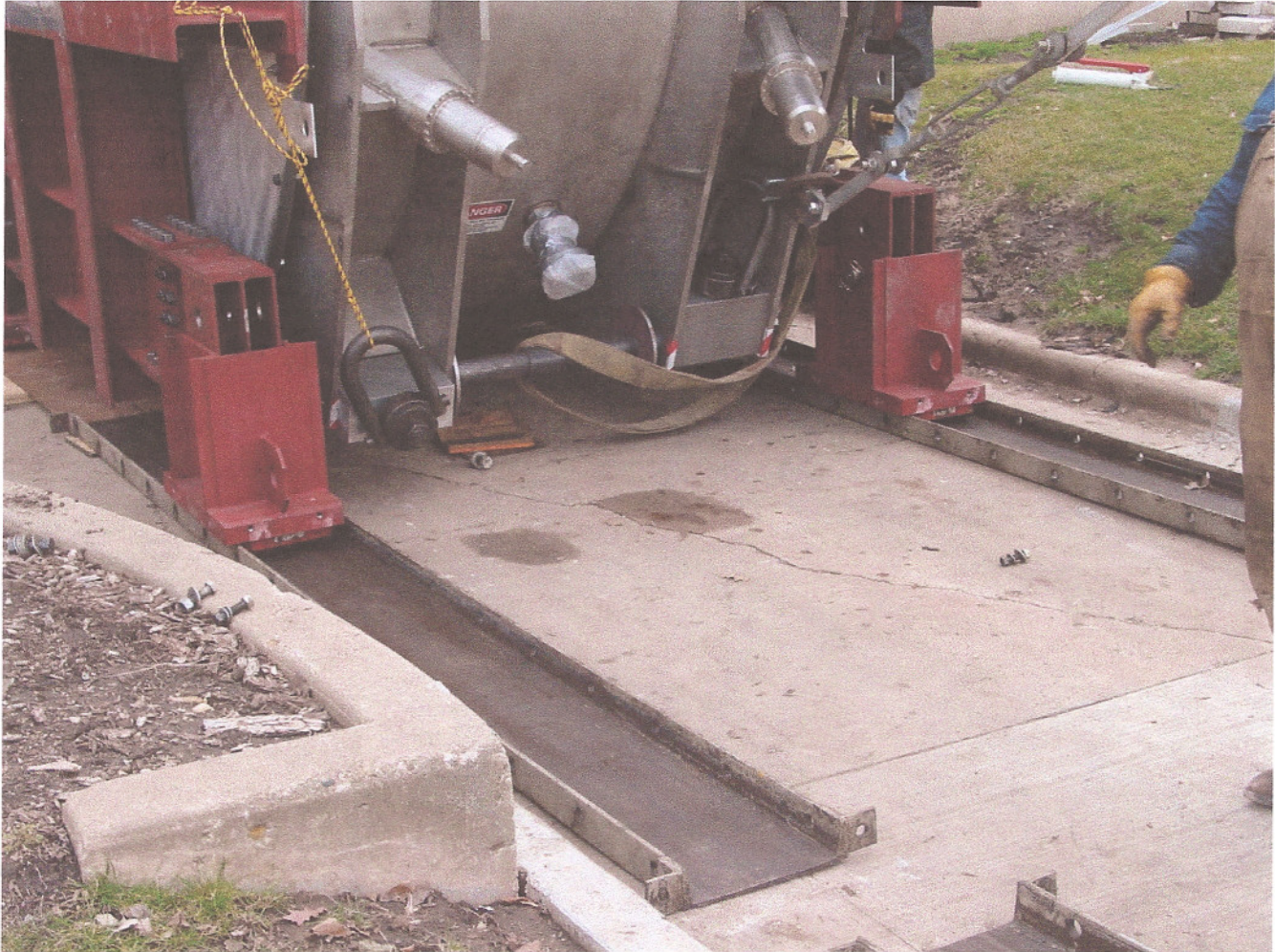
Photo 6 Going up a Ramp in Illinois with Guide Rails
